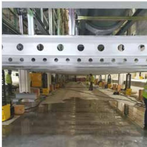
◀ Completed in just over one hour, the 160-ton 164 x 23 feet steel racking system was lifted synchronously to a height of 7.2 feet using 16 Enerpac SCJ50 Cube Jacks powered by a single SFP-Series Split-Flow Pump. Lifting large racking systems can be hazardous, complex and difficult involving forklift trucks and chain blocks. Photo by courtesy of PHL Hydraulics Ireland Ltd.
