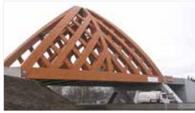
◀ Typical stage-lift application using a custom built Enerpac system to lift the 360-ton Akkerwinde wooden bridge in the Netherlands.
